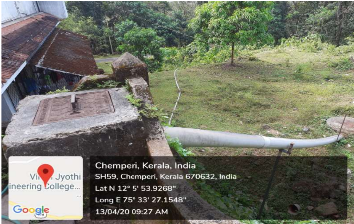
Figure: Bio gas plant near the Mess hall- feeding pipe extension point
