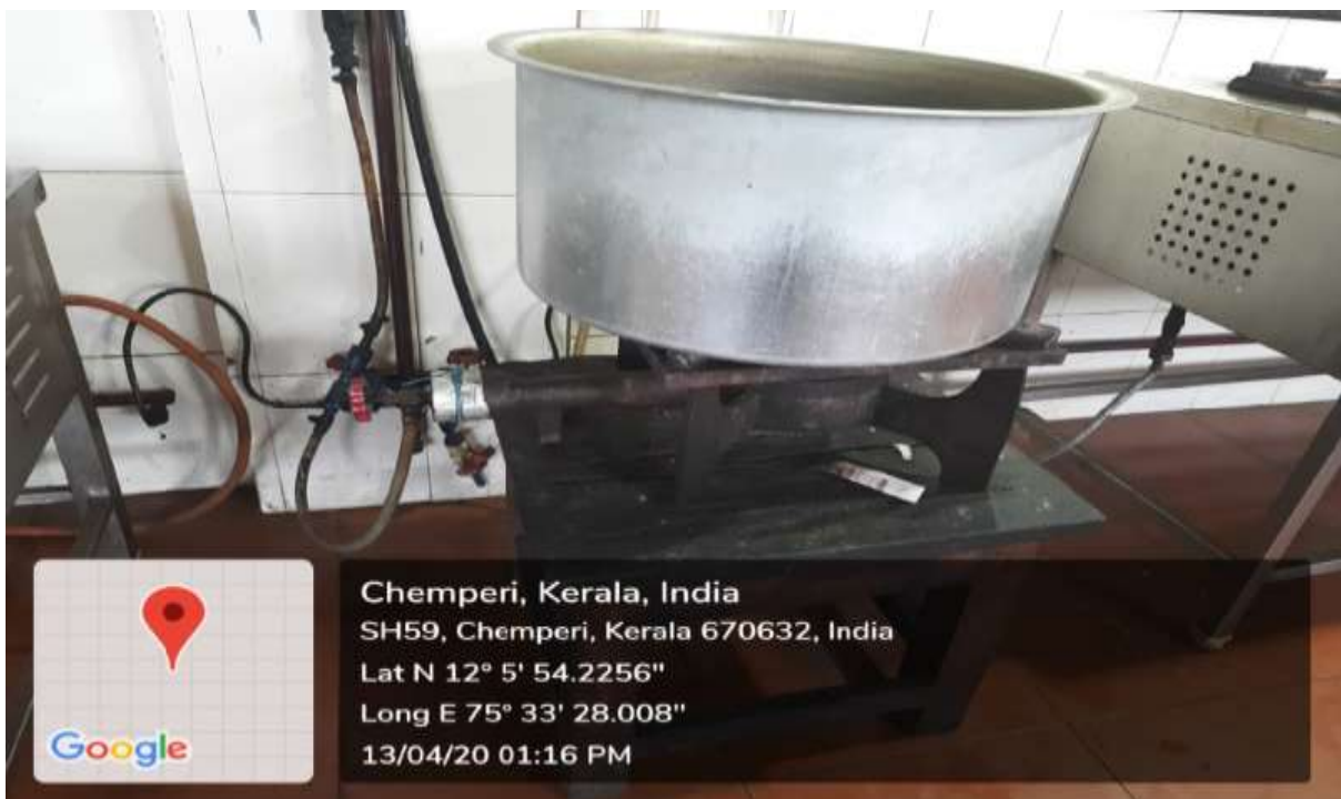
Figure: Cooking– connected with Biogas production Plant
