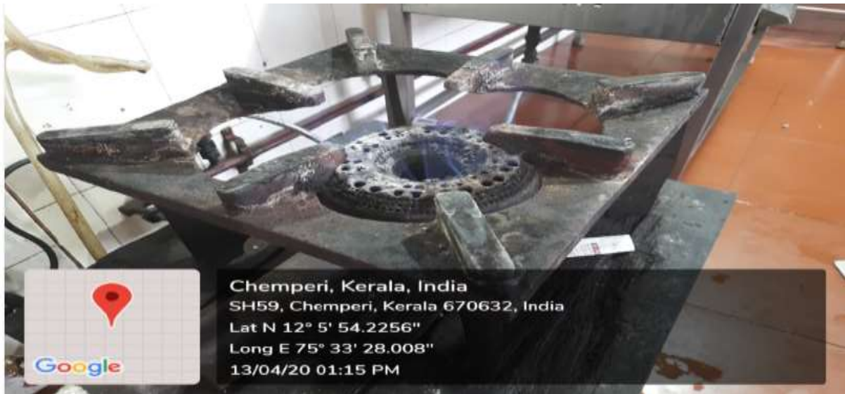
Figure: Cooking Stove burning – connected with Biogas production Plant
