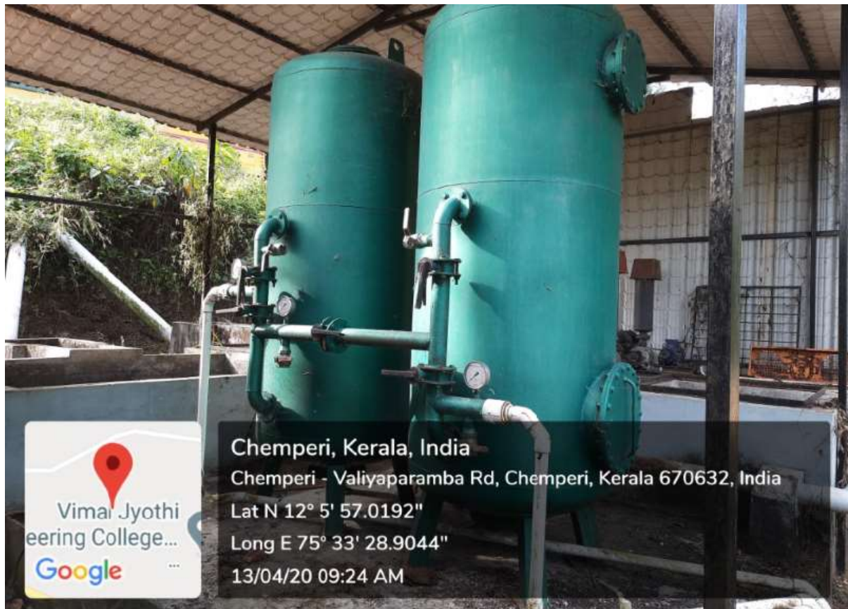
Figure: water purification and recycling units
