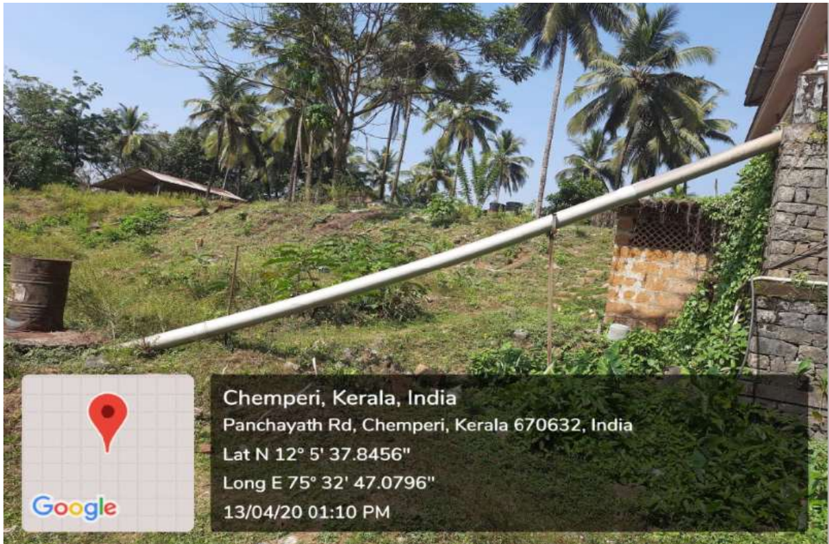
Figure: Biogas Plant- with feeder line and feeding mouth.
