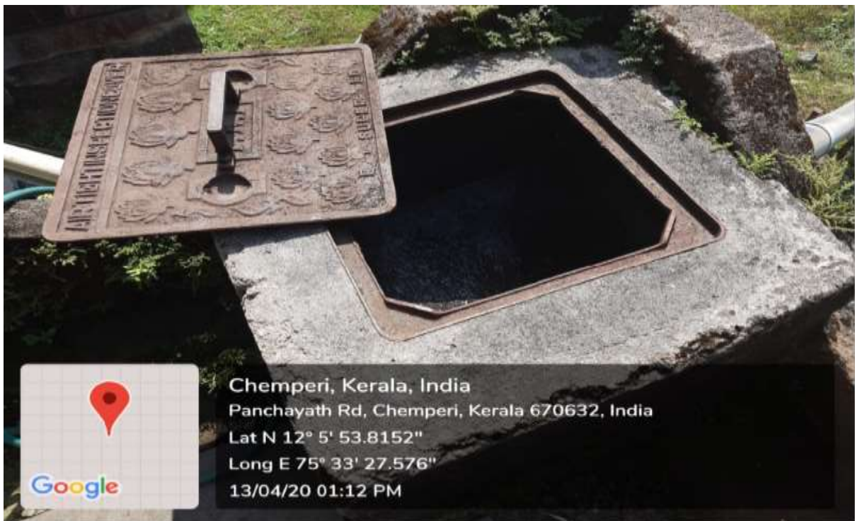
Figure: Biogas Plant- feeding mouth secured with movable lid for ease of operation- picture.
