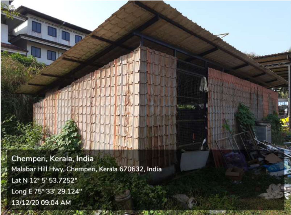
Paper waste collection and sorting centre
